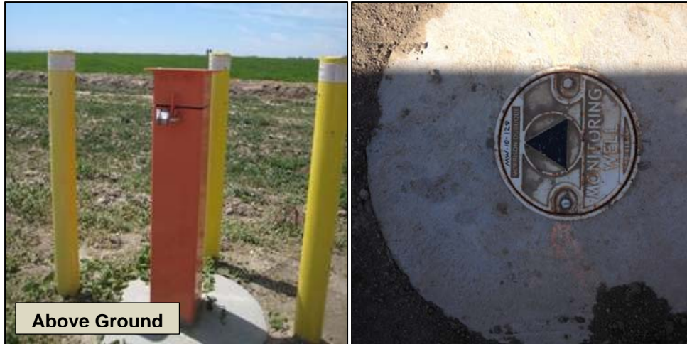
Figure E-1. Typical Construction for SJRRP-Installed Monitoring Wells
